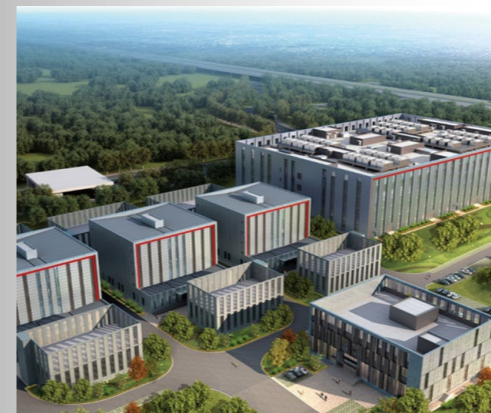
Huawei Data Center, China
